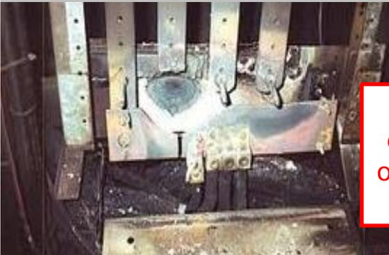
As busbar joints degrade, they can overheat and cause a fire risk.
